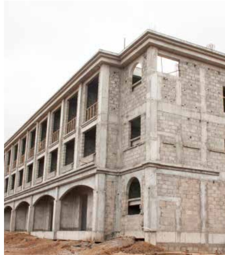
Lecture rooms during construction
